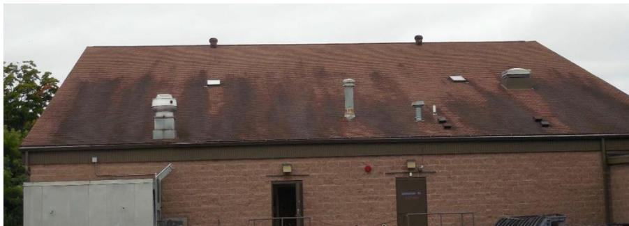
Parish Center: Shows uneven drying of roof due to ventilation and air flow issues
